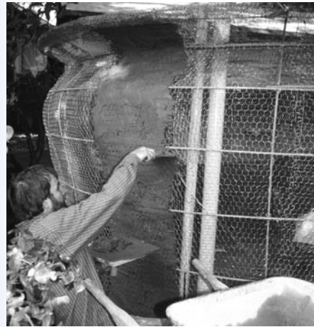
The outside and inside of the tank are hand-plastered.
