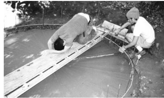
The floor is leveled to a 2 percent slope toward the drain.
