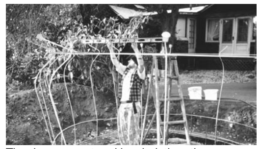
The rings are set and leveled, then the verticals placed.
