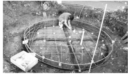
A rebar foundation grid and concrete-filled trenches reinforce the floor.
