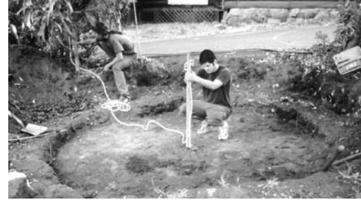
The excavation is graded for slope with a water level.
